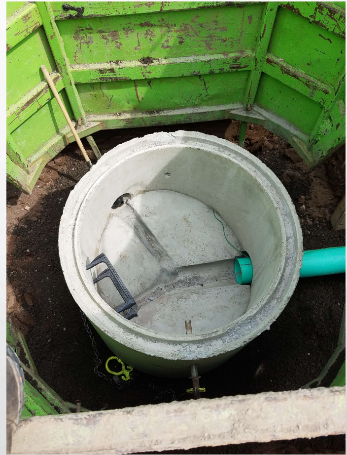
Mainline extension project
