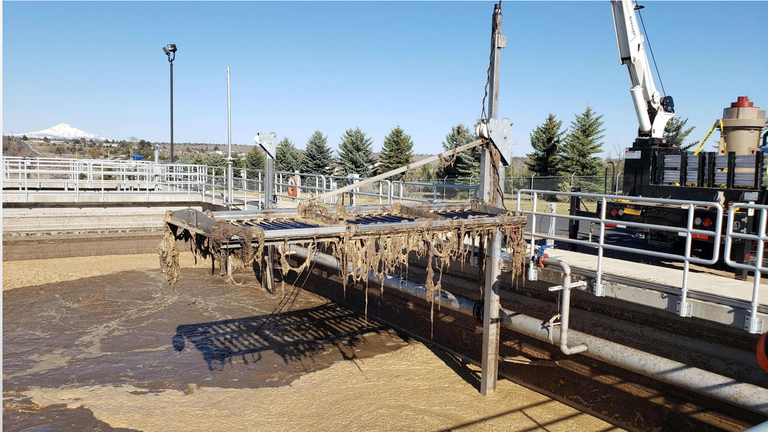
Maintenance of diffuser banks
