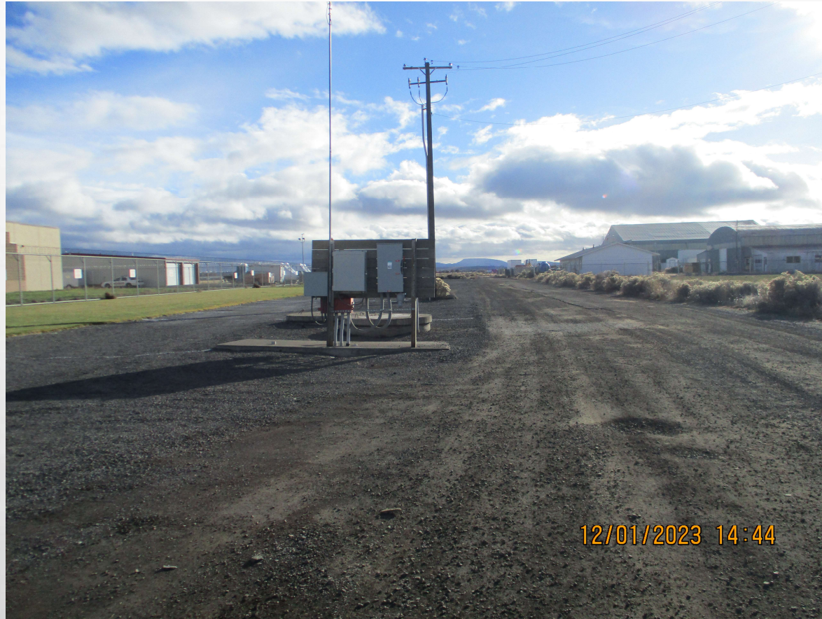
Demers pump station constructed in 1989
