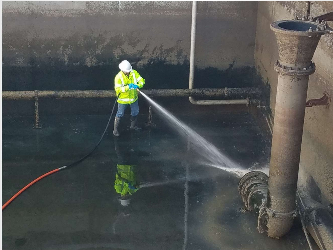
Draining and cleaning the post equalization basin
