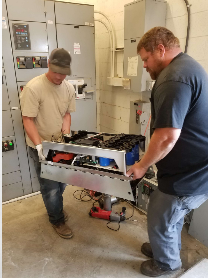
Installation of new VFD on effluent pumps
