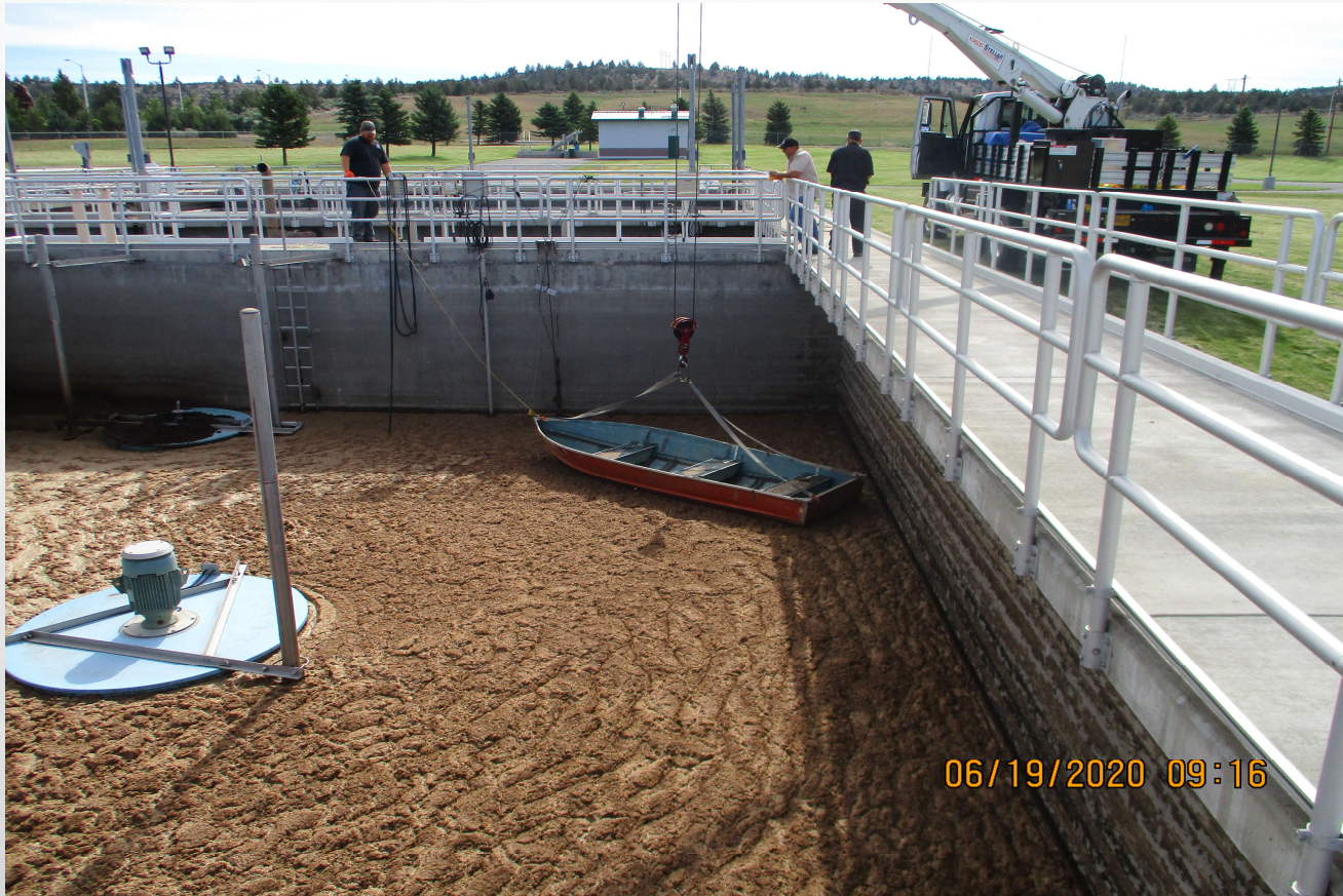
Mixer repair in the sludge holding tank (SHT)
