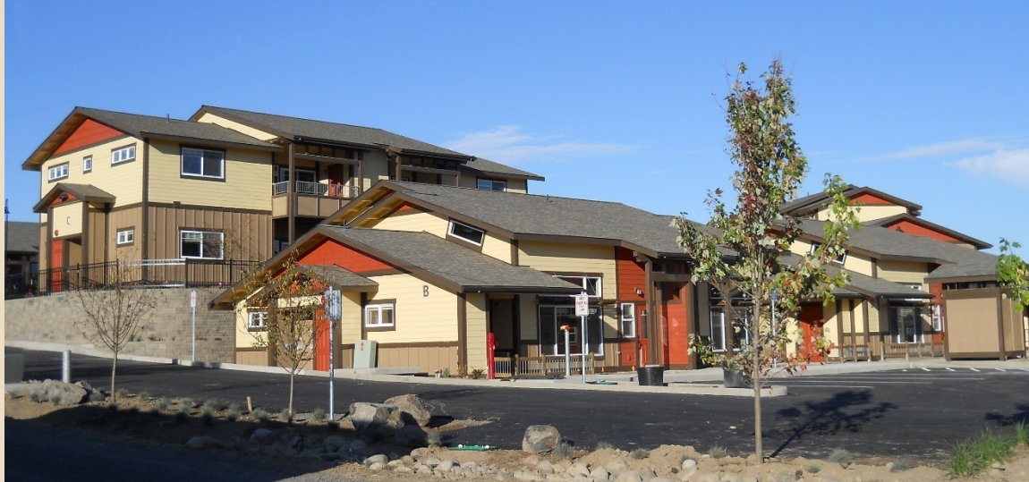
Canyon East NE Jefferson Street, Madras 24 Units Family Housing Built in 2011
