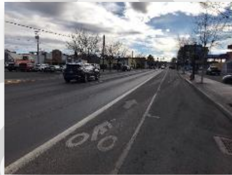
Figure Q: Madras: Bike lane – looking southbound on 4 th Street
