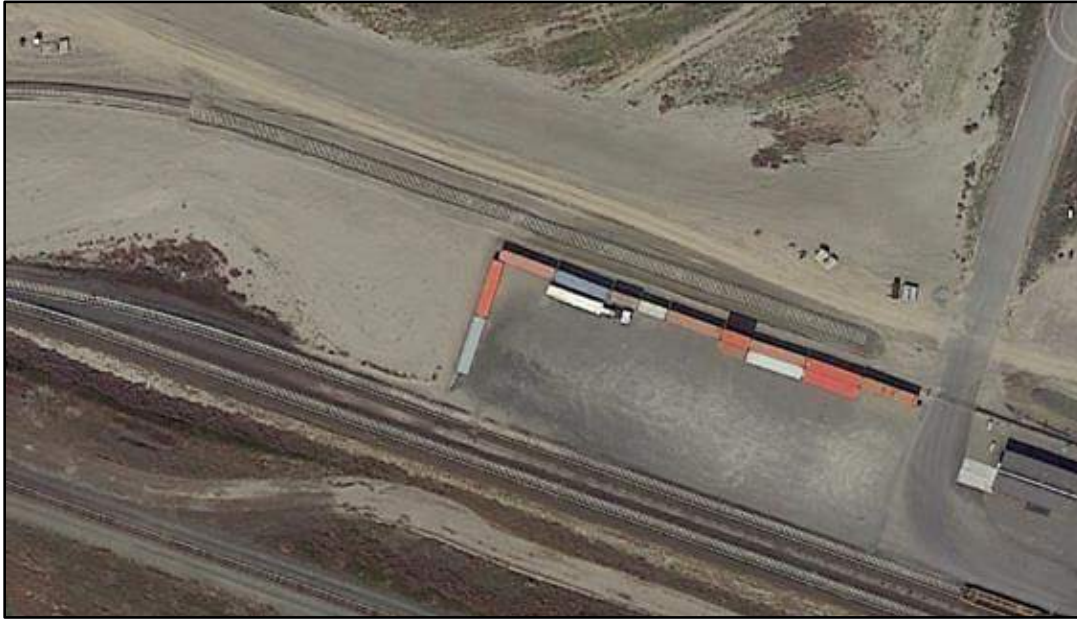
Figure 3: Recently completed intermodal facility located just east of Boardman on Union Pacific's main line (located in extreme left hand corner). Siding was constructed just off of UP's right-of-way and was paid for using the ConnectOregon funding program.
