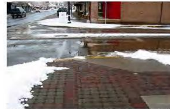
Brick pavers on 5th Street, a legacy of a past urban renewal effort
