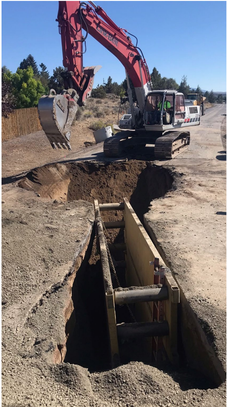
Photo: Grizzly Road sewer construction
