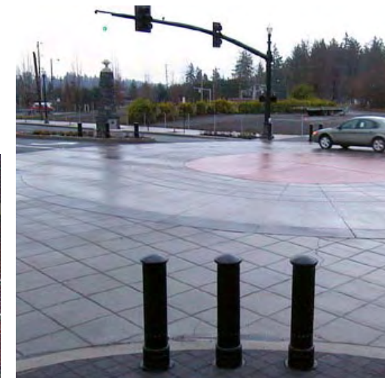
This intersection in Lake Oswego has been repaved, creating a signature gateway, slowing car traffic and making pedestrian crossings safer. Note the bollards separating the roadway from the sidewalk.
