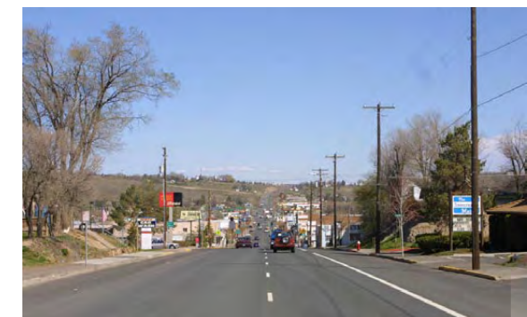
Northbound US 26/97. The width and speed limit of this roadway encourages speeding and discourages walking.
