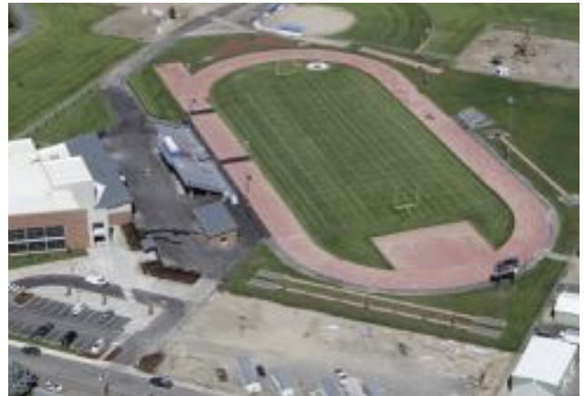
Madras High School New Recreational Facilities
