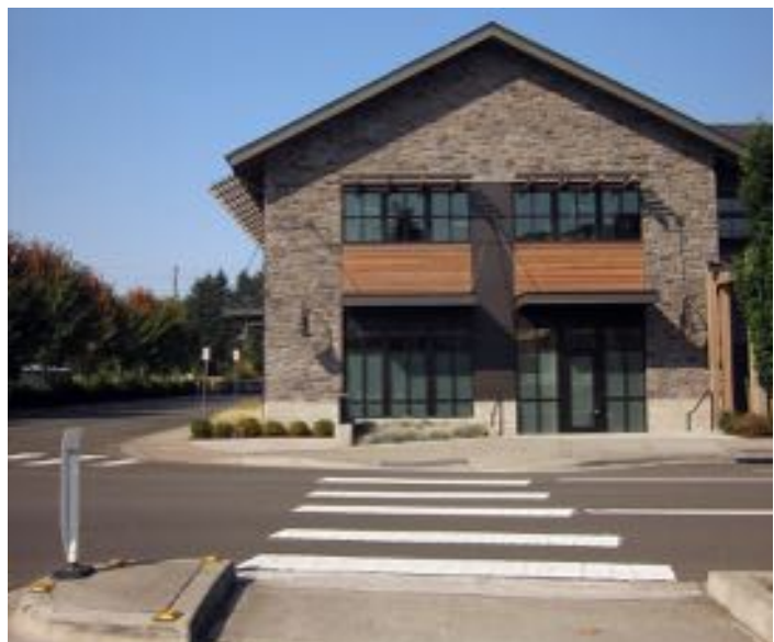
The aesthetic of new office or retail spaces can reinforce and strengthen the character of downtown Madras
