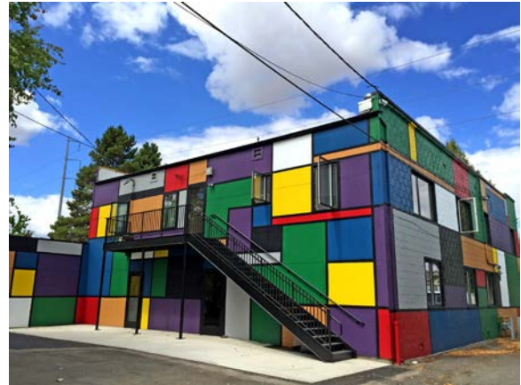
Second Floor Office Space in Concrete Block Bldg
