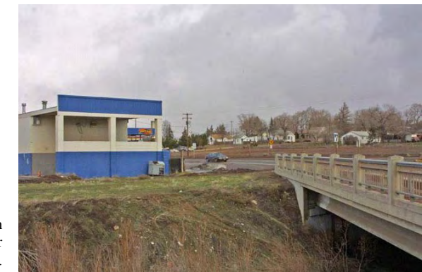
View A on sketch above. North bank of Willow Creek near southbound bridge of US 26/97.
