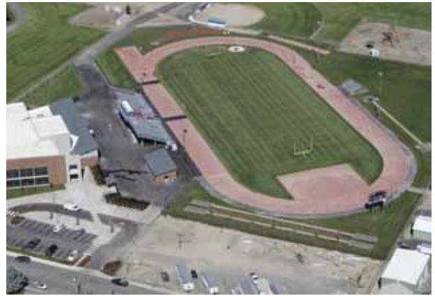
Madras High School New Recreational Facilities
