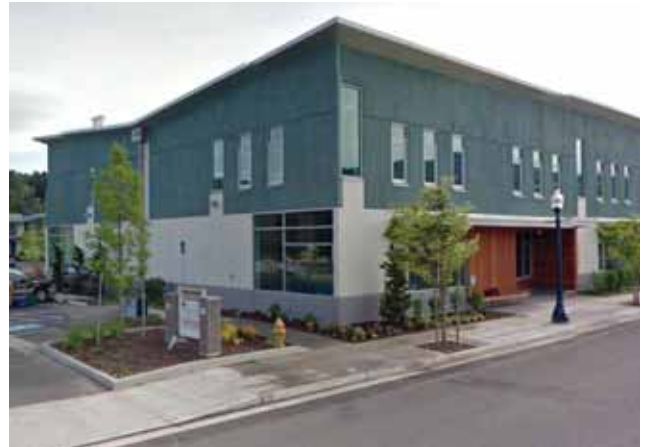
Brewery building with attractive streetscape
