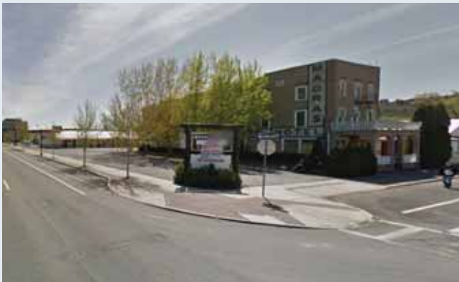
Existing Madras Hotel Motel at SW C Street and SW 4th Street
