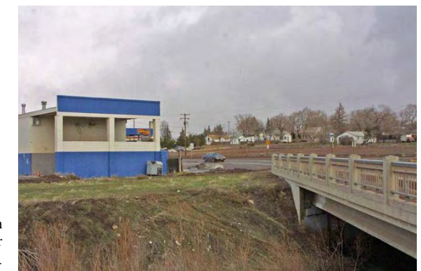
View A on sketch above. North bank of Willow Creek near southbound bridge of US 26/97.
