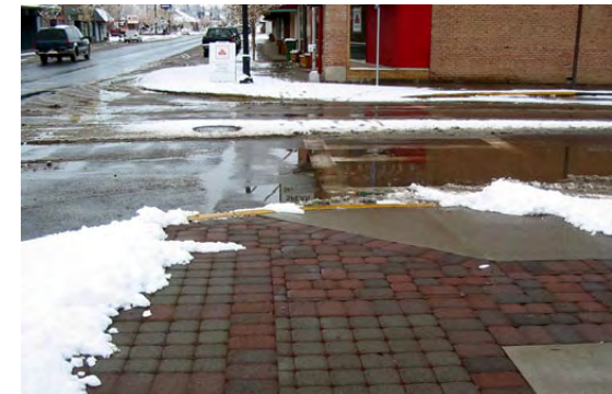
Brick pavers on 5th Street, a legacy of a past urban renewal effort
