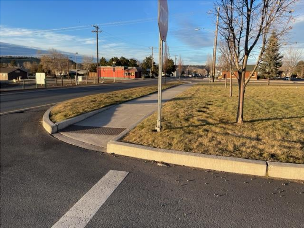
Figure 7. Applicable AASHTO Sight Triangle view toward the north at the US 97 Southbound/Prince Place intersection.
